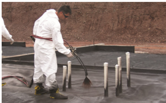
Figure 11. Spraying an emulsified asphalt latex barrier.
