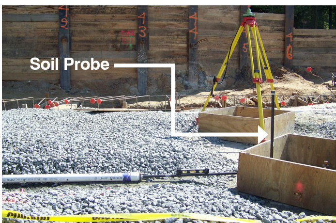
Figure 13. Forms for vertical column support pad with embedded soil probes.
