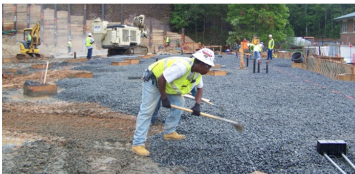
Figure 2. Proof-rolled ground covered with 8 inches AASHTO #57 stone.
