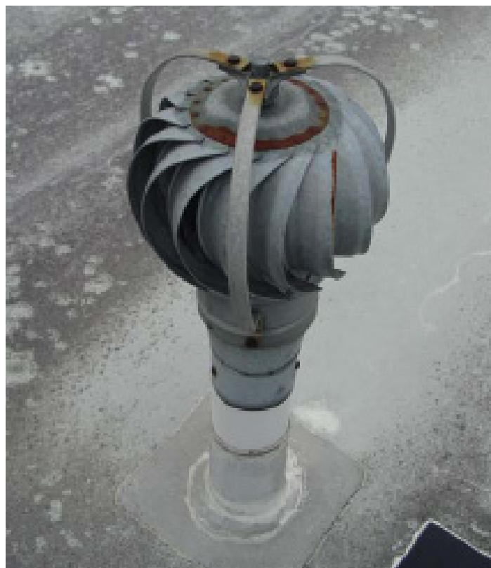
Figure 16. Roof vents fitted with wind turbines provide slight depressurization of the sub-slab area and prevent the buildup of contaminants beneath the building.
