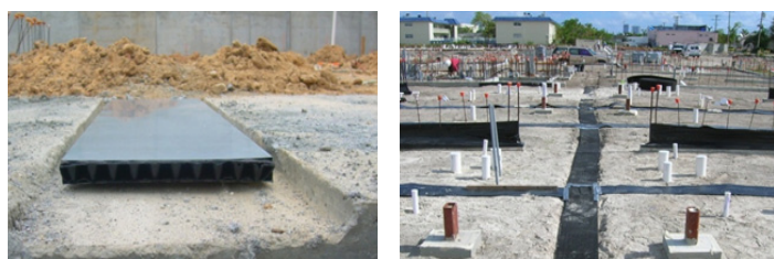
Figure 6. Commercial venting product has properties similar to 4-inch PVC pipe with lower installation costs.
