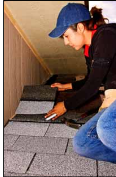
A Texas Bootstrap Loan recipient places a roof shingle into place.
