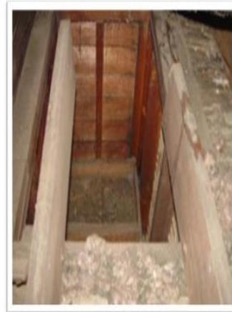
Use any air-barrier (sheetrock, foam board, plywood, etc) cut to fill in the area and foam seal in place.
